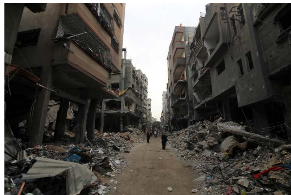
Figure 19: Destruction in Al-Shati refugee camp, Gaza Strip (29 October 2023). Photographer: Mohammed Zaanoun.
