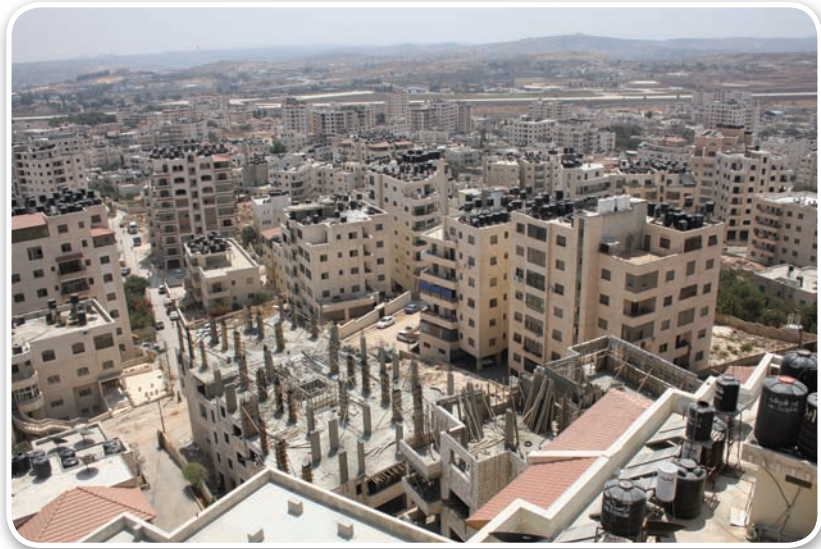
Construction boom in Kufra Aqab. August 2010 - © Al-Haq
